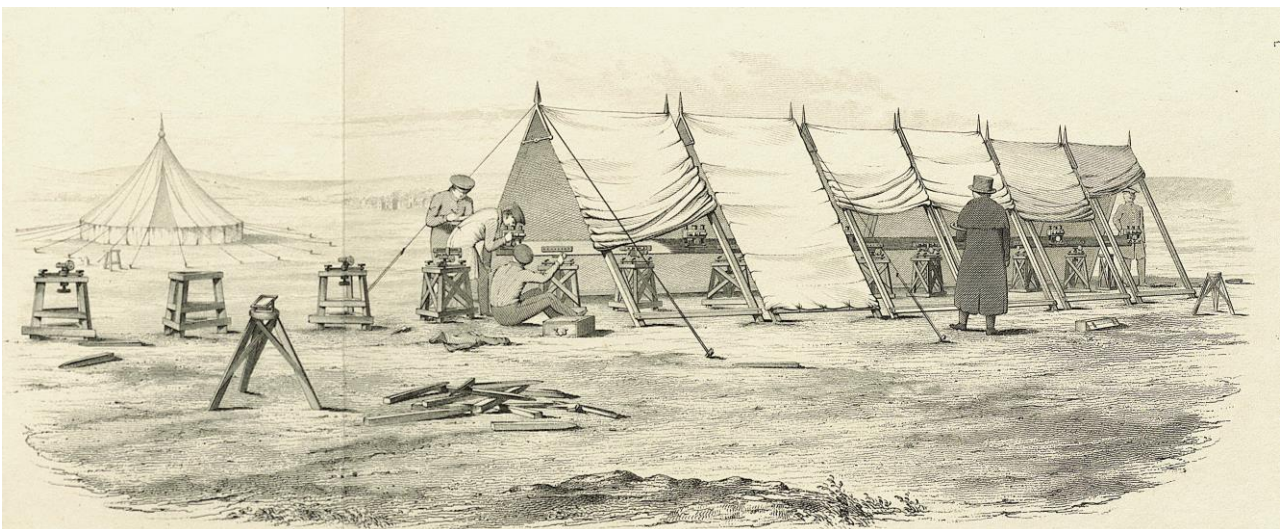
Figure 6. Engraving of a sketch made by Sir John Herschel when visiting the baseline, showing the tents covering the compensating bars laid out for measurement.
