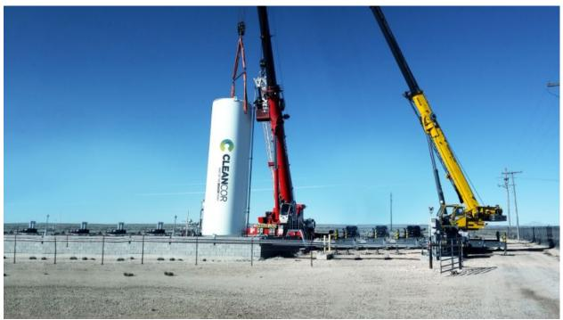
Properly positioning an LNG storage container at a permanent asphalt production facility can be scheduled over a weekend to minimize plant downtime. Photos courtesy of CLEANCOR
