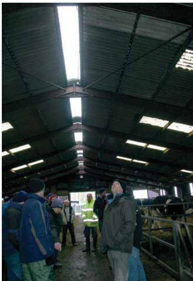
Bull finishing shed – after ridge removed
