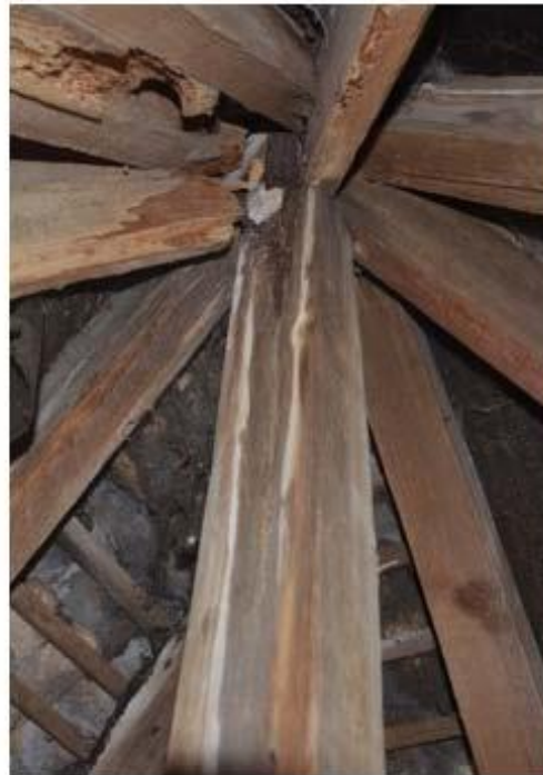
Fig.2: Extent of rot to roof apex
