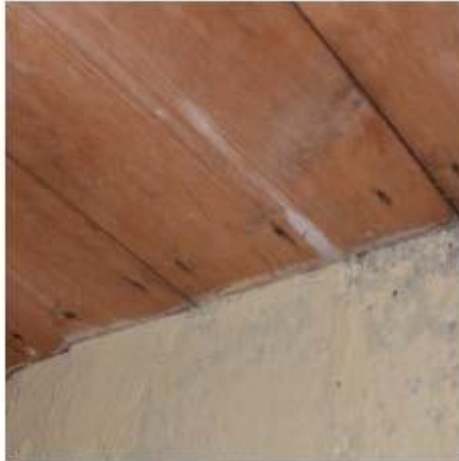
Fig. 7: Evidence of leaking on ringing chamber ceiling
