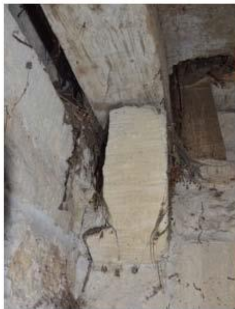
Fig. 6: Spalled corbel stone
