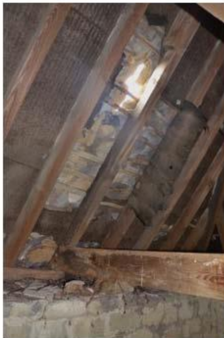
Fig.1: Leaking roof on the South quadrant
