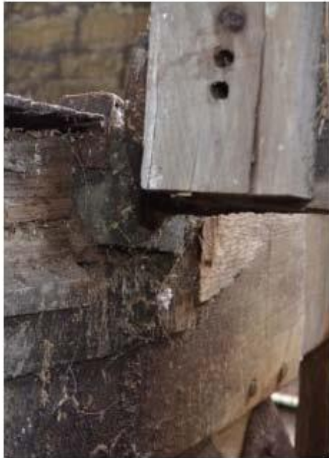
Fig. 3: Damaged bell frame below Second strap gudgeon
