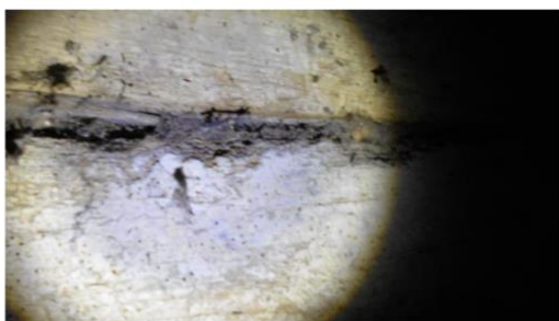
gaps in timbers of first floor with cobwebs and nesting debris
