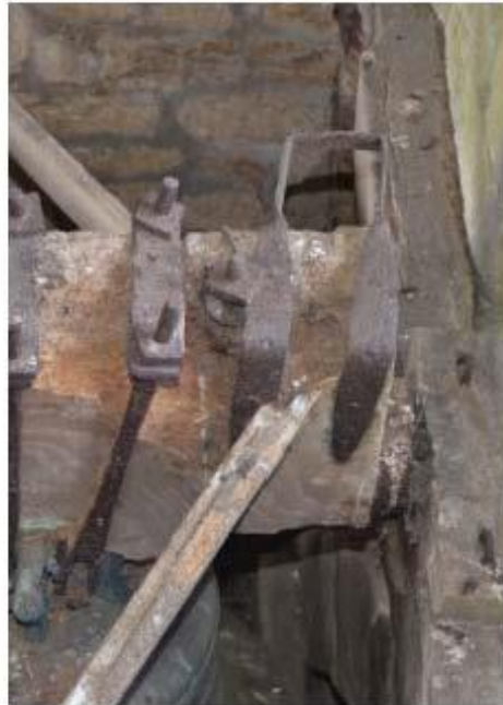
Fig. 4: Extent of rot to Treble headstock
