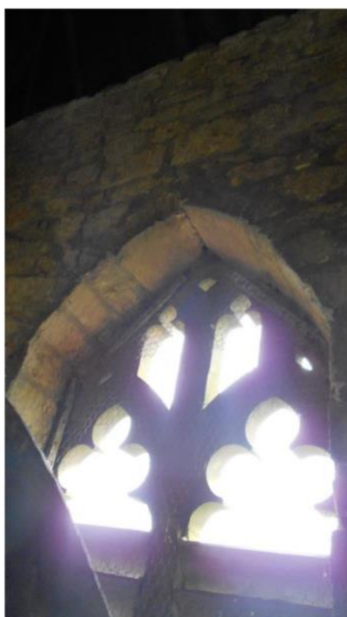
second floor window with missing wire mesh
