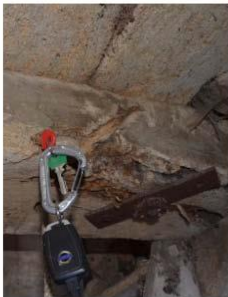
Fig. 5: Extent of rot/decayed knots to Treble support beam
