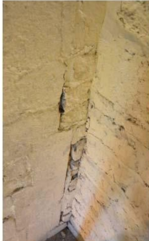
Fig. 8: Loose mortar around window infill on East wall of ringing chamber
