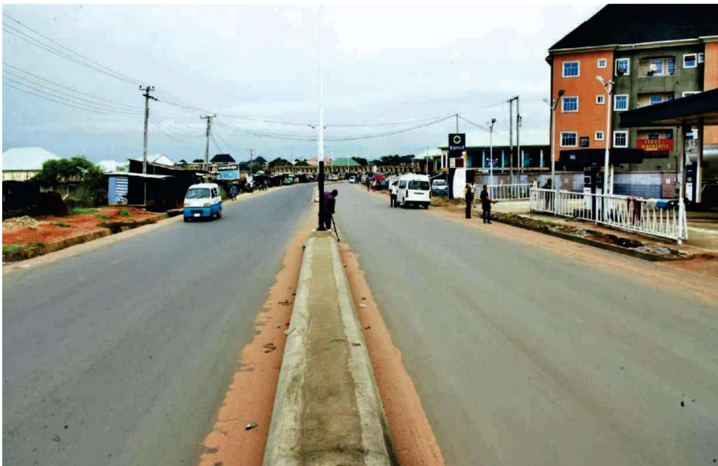
RECONSTRUCTION OF OWERRI-ORLU HIGH WAY
