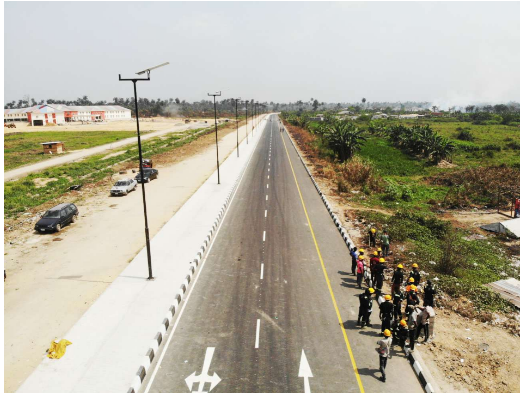
AIT/IGBOGENE ROAD COMPLETED
