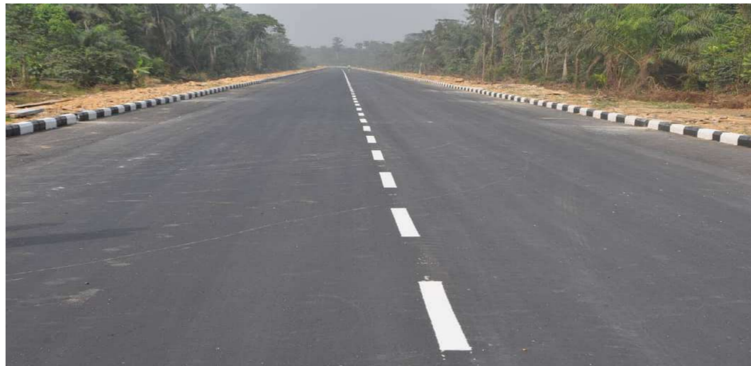
IGBEDI ROAD COMPLETED
