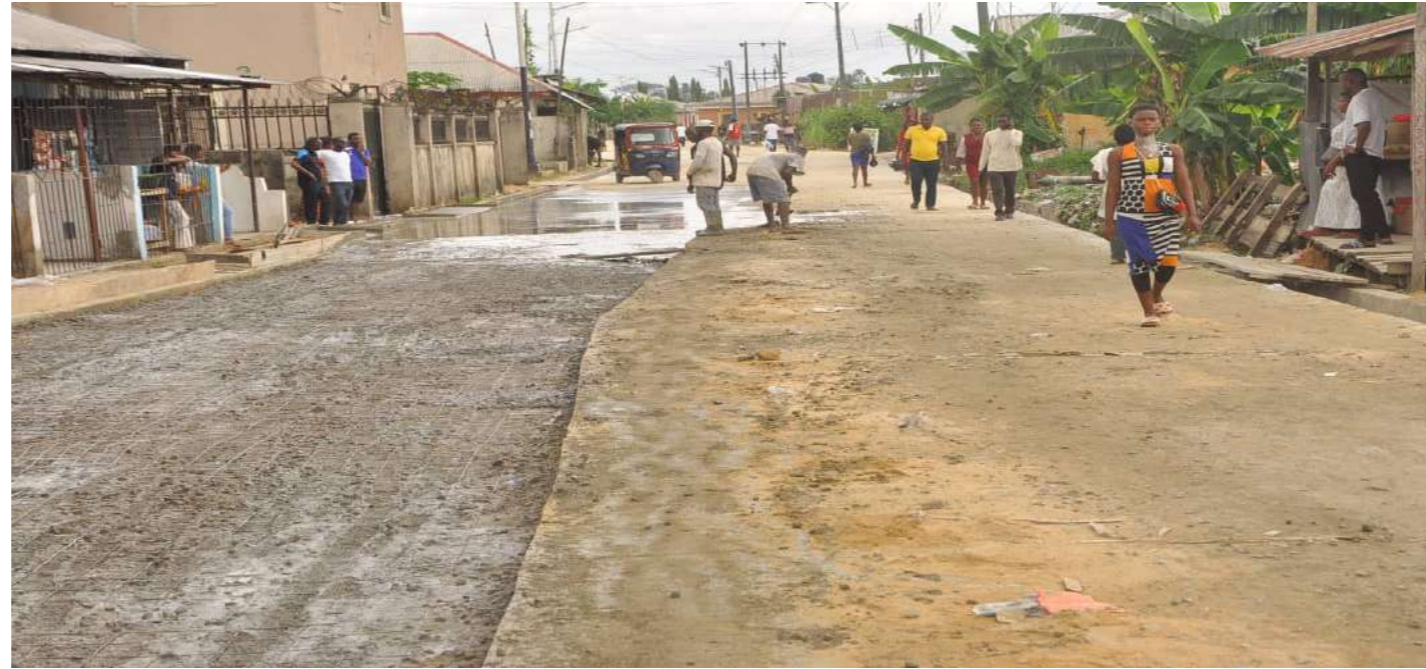
ROYAL FM ROAD ONGOING
