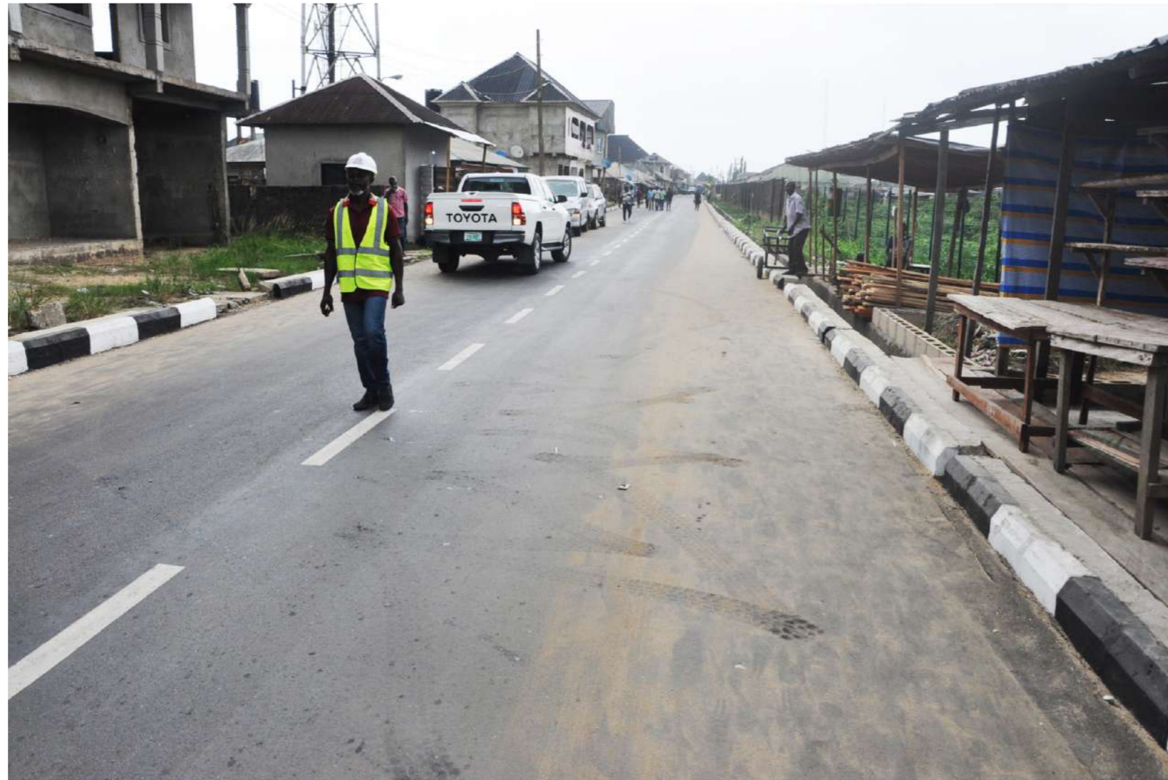
LAW SCHOOL ROAD COMPLETED
