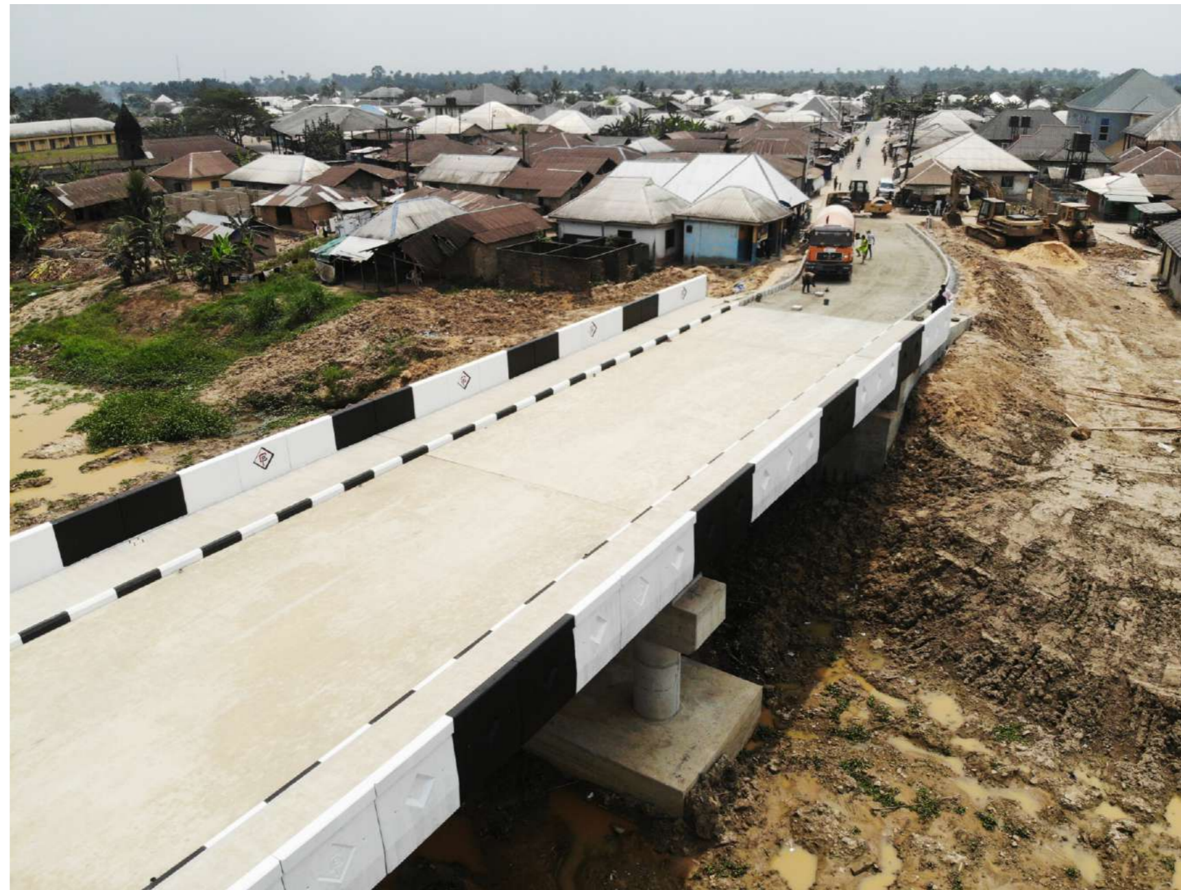
ELEBELE BRIDGE COMPLETED
