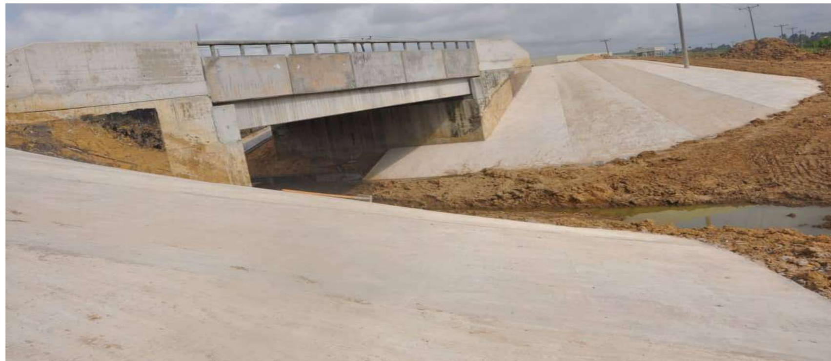
SAGBAMA/ EKEREMOR ROAD PHASE 1 COMPLETED
