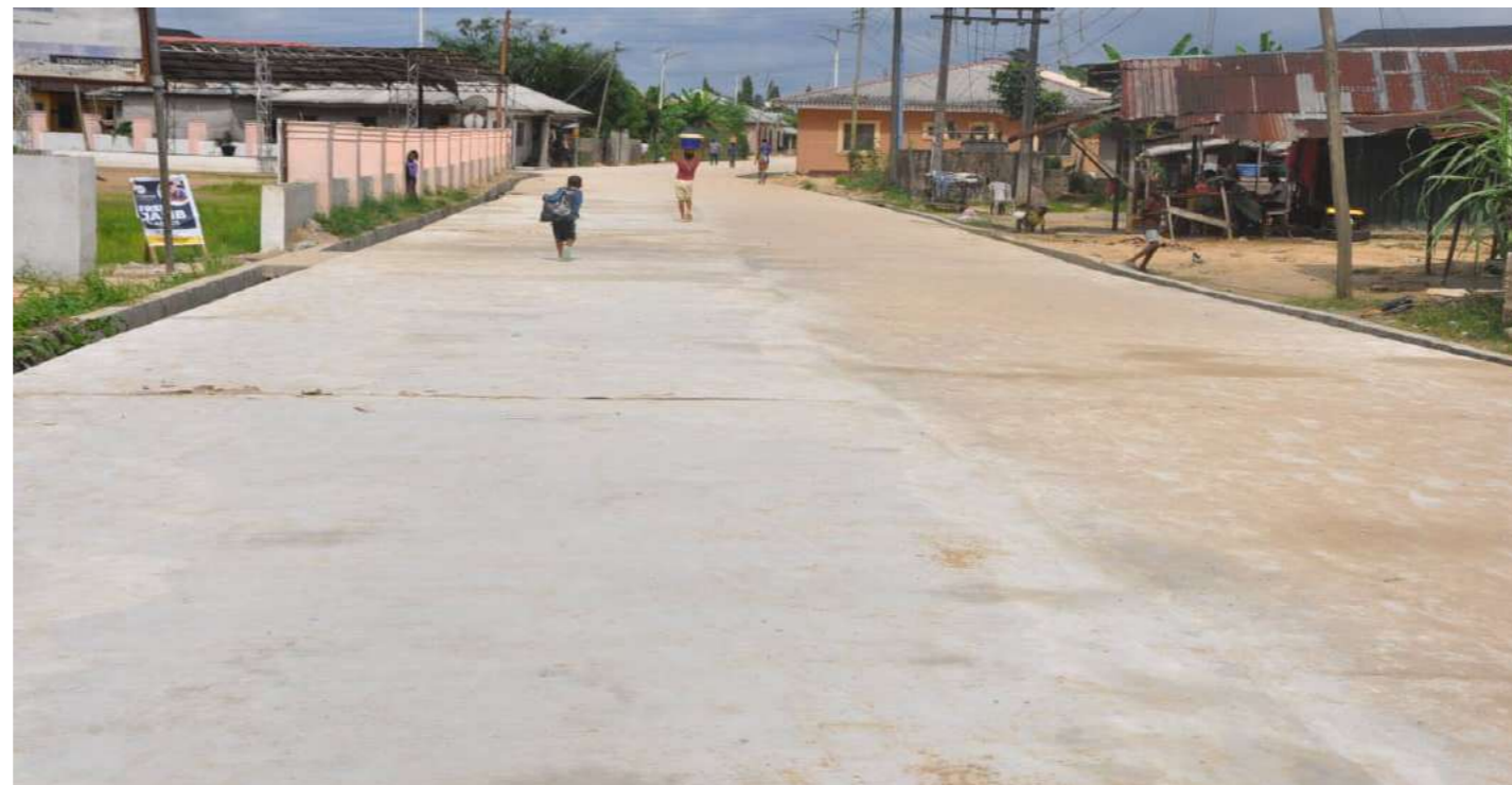
ROYAL FM ROAD COMPLETED
