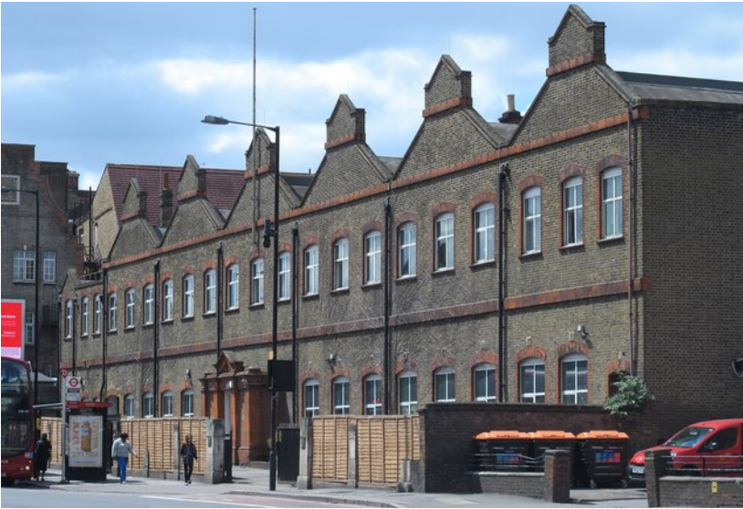
Ivy House, Hackney ©Morris+Company
