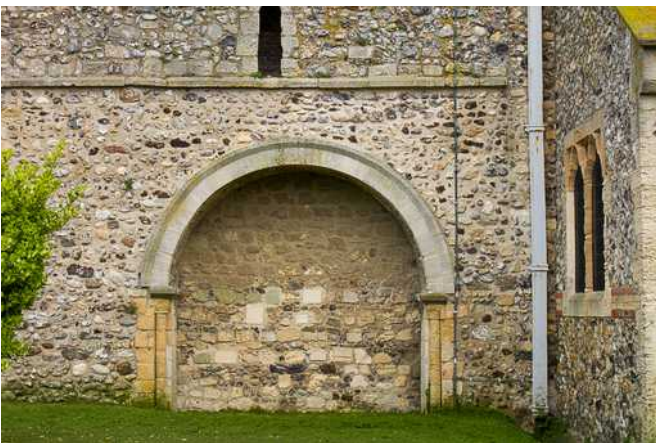
12 th Century Caen stone arch (with repaired facing?) in the south side of the tower of St. Leonards Church, Seaford.
