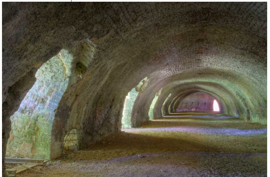
Hoffman kiln, Llanymynach. Although this example was a lime kiln, the same design was used to fire bricks. Photo ©Richard Becker.
