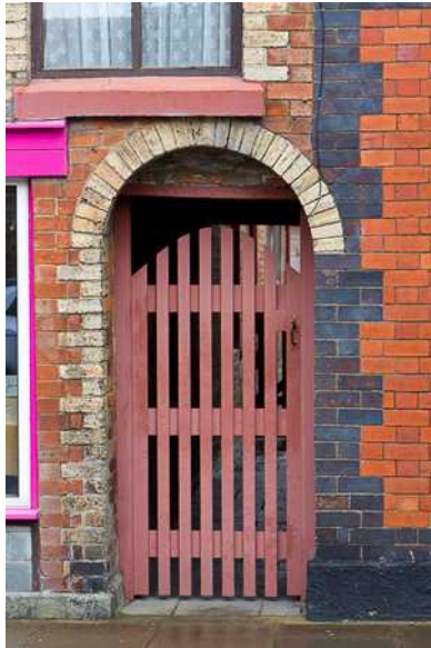
Polychrome effect from coloured bricks on adjacent houses. Short Bridge Street, Llanidloes. Photo ©Richard Becker.
