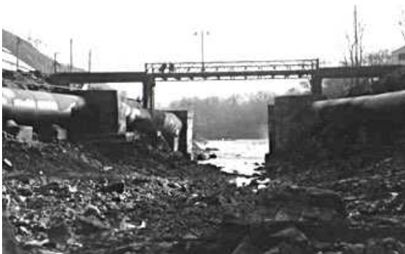
The Bailey Bridge access to the north bank.
