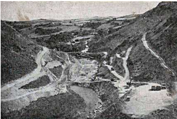
The excavations have started.
