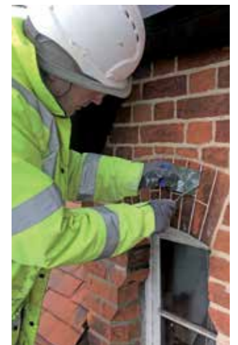
■ Decorative 'tuck-pointing' to brick arches of the Caswells' House Room windows.
