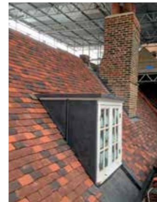
■ Before and after views showing the Front Quad side of the library roof. The dormer windows in the library roof have had new traditionally detailed casements fitted. The tops and sides of the dormers are clad in lead work.
