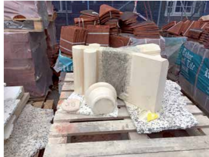
■ High-level stonework had badly eroded, in this case a finial cross from the gable end of Lambourne's and Caswalls' House Rooms, seen here awaiting re-installation following repairs.
