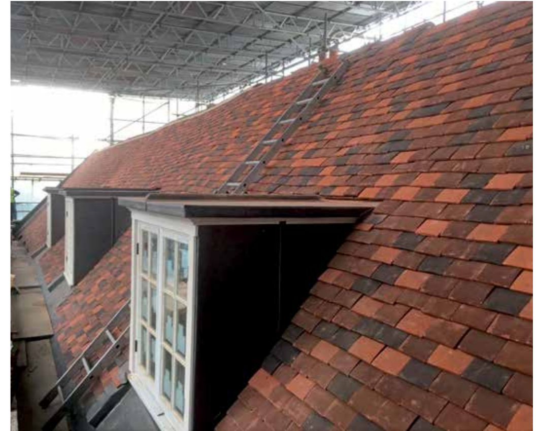
■ Before and after views showing the Front Quad side of the library roof. The dormer windows in the library roof have had new traditionally detailed casements fitted. The tops and sides of the dormers are clad in lead work.
