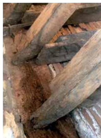
■ Front Quad before the work started. From ground level the extent of roofing defects was not immediately apparent, but the buildings had a decidedly tired appearance. The roof above the library was the highest priority area, but despite decay in the rafter-ends caused by long-standing roof leaks, the majority of the 400-year-old oak framing remained in good condition.
