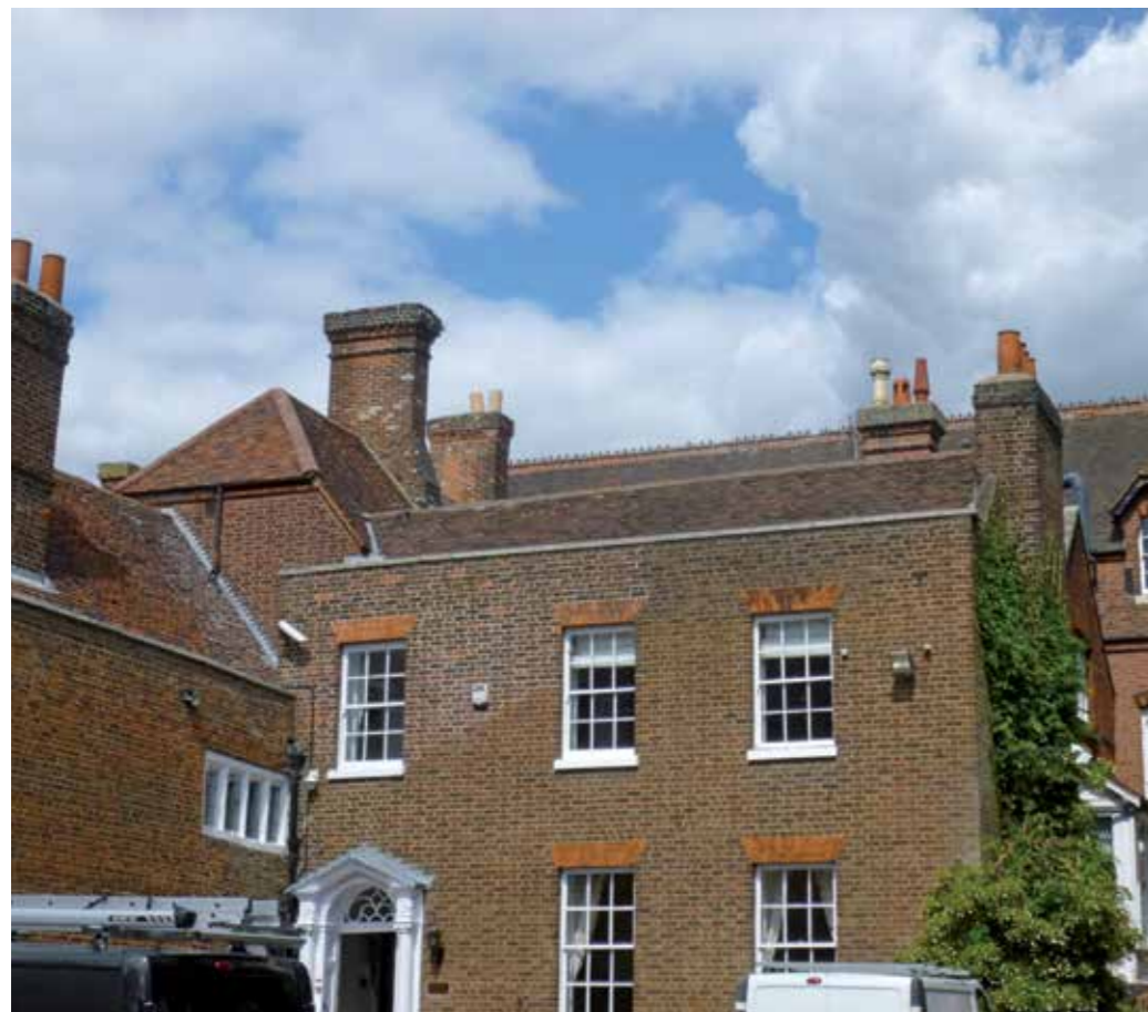
■ Front Quad before the work started. From ground level the extent of roofing defects was not immediately apparent, but the buildings had a decidedly tired appearance. The roof above the library was the highest priority area, but despite decay in the rafter-ends caused by long-standing roof leaks, the majority of the 400-year-old oak framing remained in good condition.
