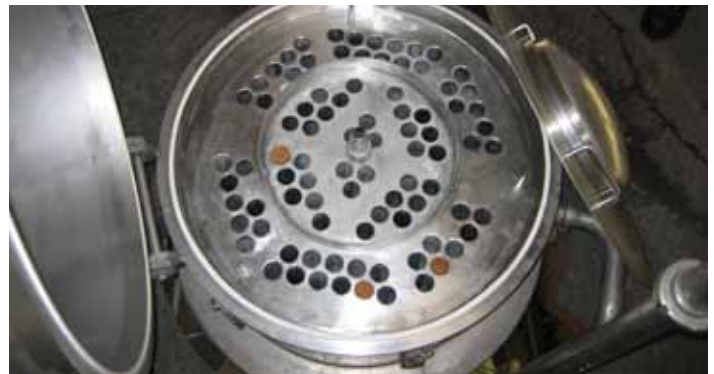
Heat Exchanger tube internals cleaned and polished for IRIS inspection
