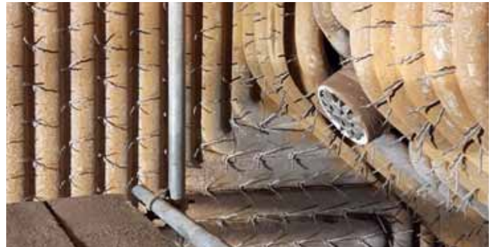
Refractory removed from boiler tubes using water jet
