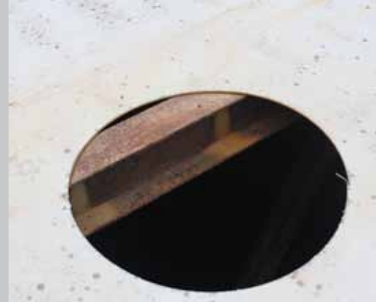
Hole cut in Gas Holder Crown using RGL's "Jetnife"
