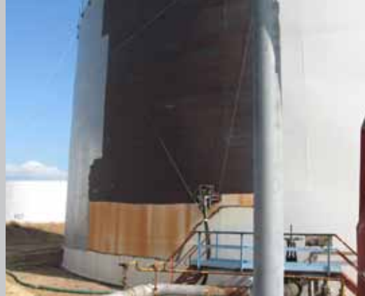
Coatings removed without scaffolding using RGL's "Limpet Crawler" vacuum blast head
