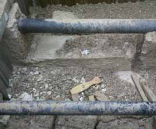
Concrete removed by water jet from around pressurised Pumping Mains
