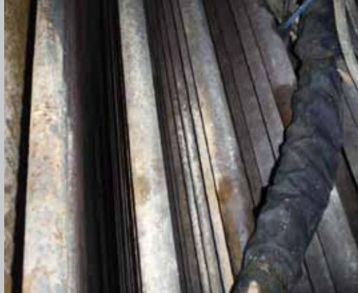
Boiler Tubes cleaned by remote control water jet
