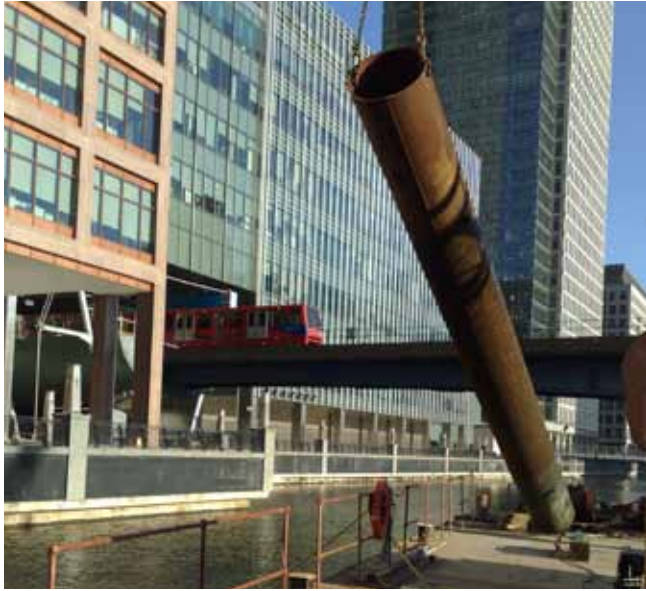
Cut pile being laid down for safe transportation
