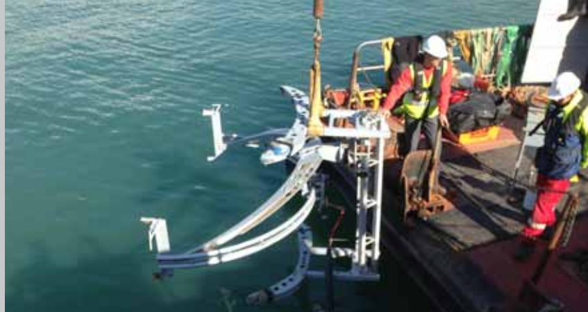
External cutting tool being deployed
