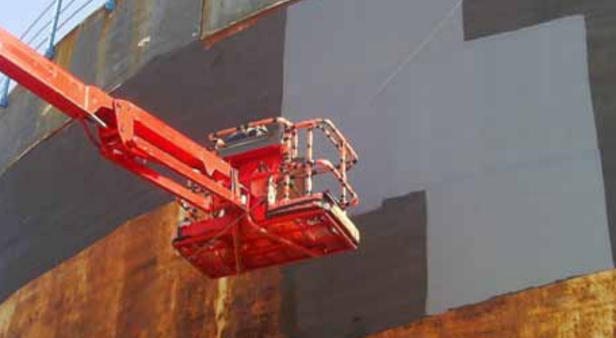
Access via MEWP for spotting & paint application
