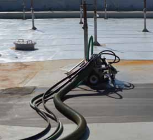
Surface preparation of floating tank roof
