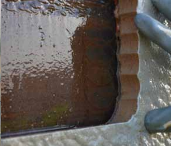
Thick coatings & insulation removal
