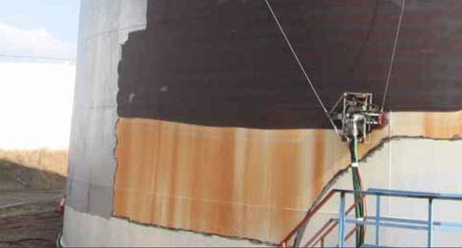
Tank side sheet preparation
