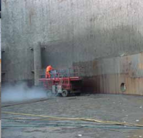
Tank lining removal
