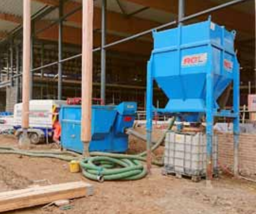
On-site set up: jetting unit, VAC power pack & hopper
