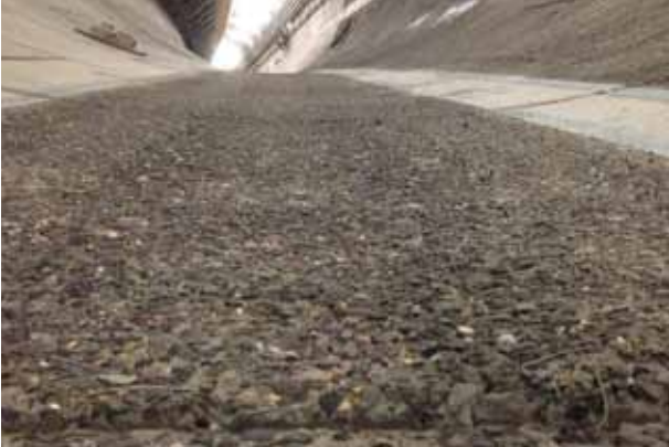
Pre cast tunnel section scabbled finish close up
