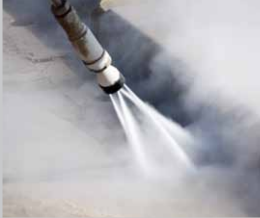
Hand held treatment with spinning UHP water jet
