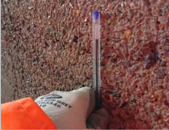
Hand held lance finishing around edges & columns
