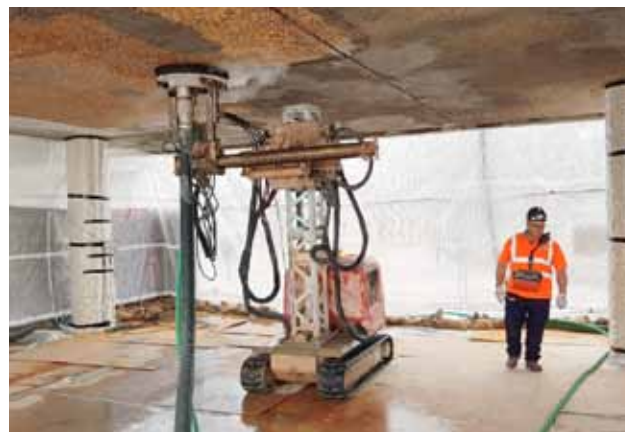
Powerful vacuum reduces noise and enables containment and recovery of waste water and concrete
