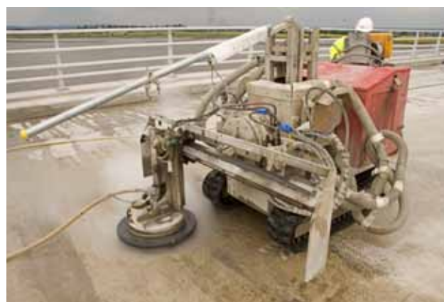
Robotic concrete bridge deck surface preparation
