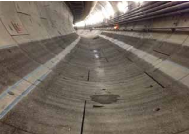
Producing a light scabbled finish on the pre-cast tunnel lining
