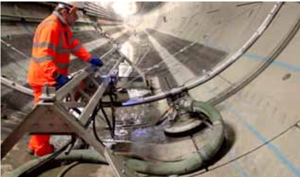
Robotic water jet scabbling for the London Crossrail Tunnel project
