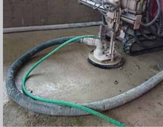
Powerful vacuum recovers waste water & debris
