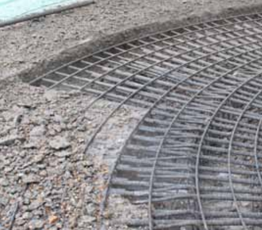
Precision concrete hydrodemolition
