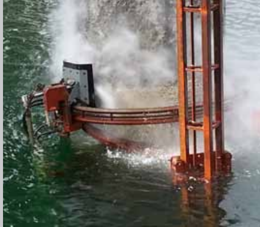
Cutting above and below water line
