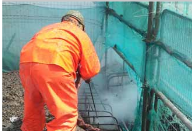
Hand held precision hydrodemolition
