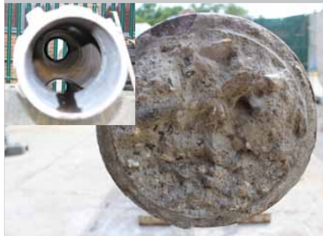
Concrete removal from blocked augers
