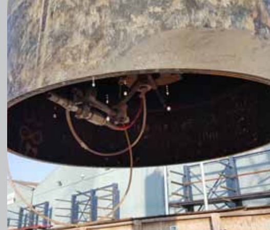
Internal steel pile cutting underwater
