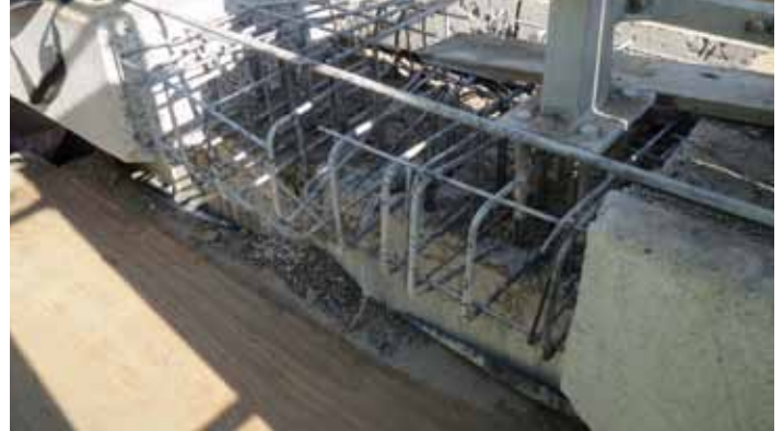
Precision cutting to create pockets on bridge parapet
