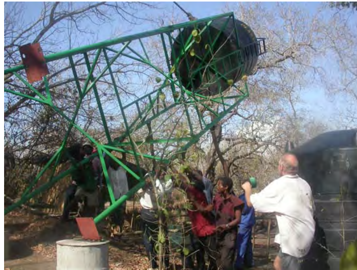
Figure 8. Erecting water tanks for the borehole.
