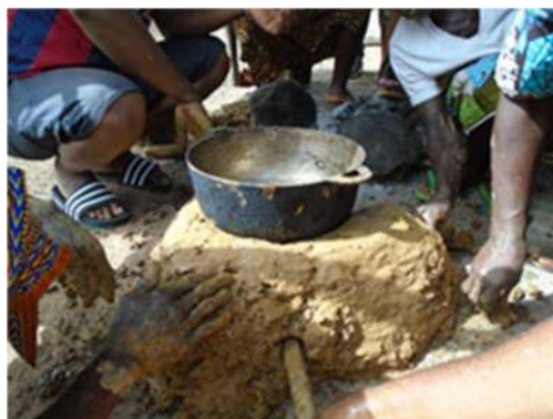
Preparation of Improved Cooking Stove that saves 10 fuel woods per day from being cut
