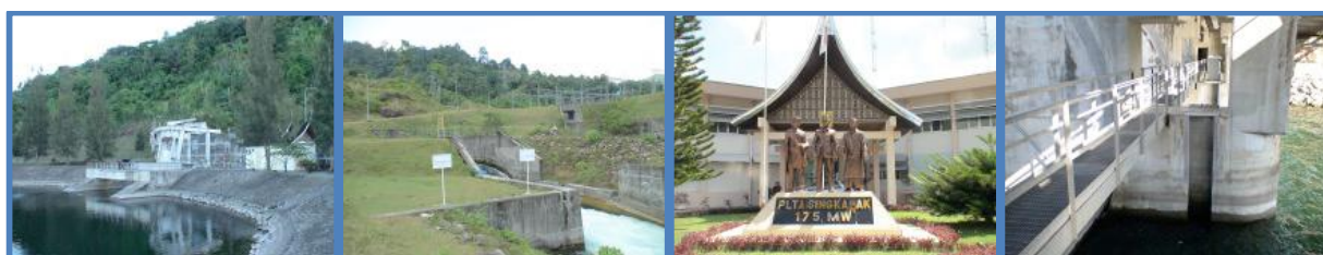
The water inlet (left), leading into a 16,500 m long headrace tunnel to the PLN power station.
