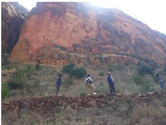
Photo 8: Stone bund constructions in Adienkrti.
