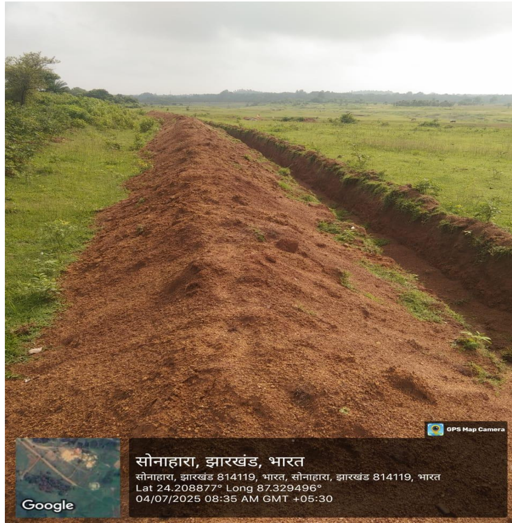
Figure 14: Cattle Proof Trench (CPT) as barrier
