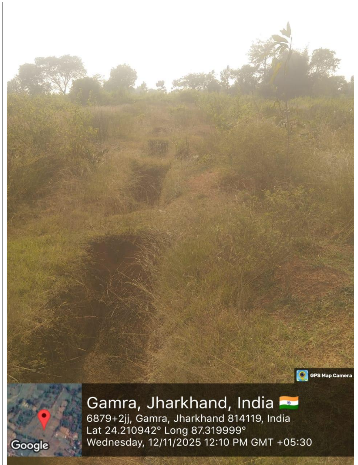
Figure 16: Staggered trenches for protection
