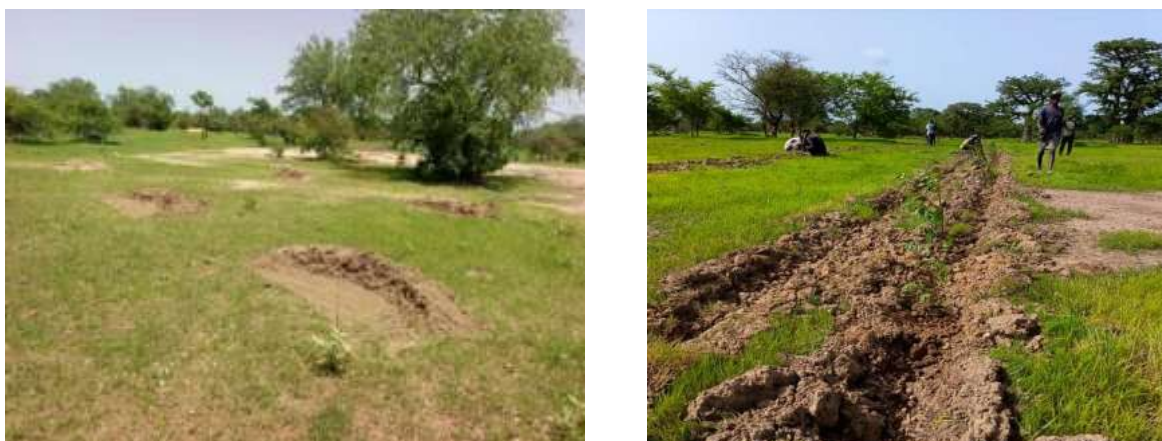
Picture 4: Example of demi-lunes constructed in planting sites by the members of the community (left) and construction of pits produced by a tractor (right).
