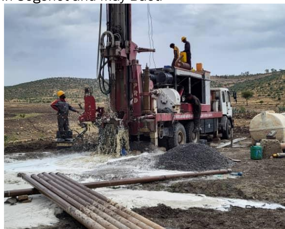
Excavation of borehole for drinking water in Amanit
