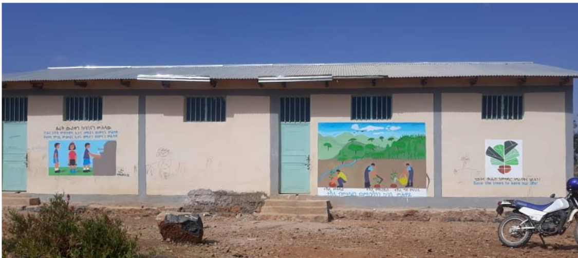
New Classroom constructed at tabia Mahbresilasse ,waseya Primary School
