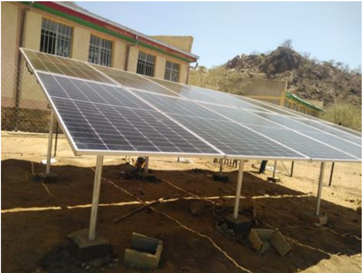
Installation of Solar energy at kolatemben, Arena Secondary school
