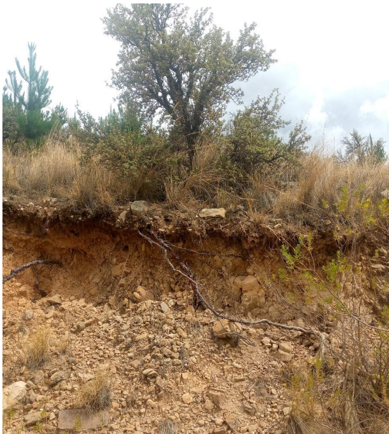
Figure 4: (above) Gullying in project area Yanarumi, 2022; (below) Pedestal erosion in project area Sub Central de Izata, 2022.
