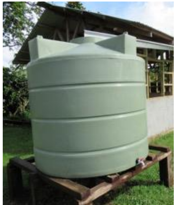
FIGURE 1 Water tank bought with carbon income
