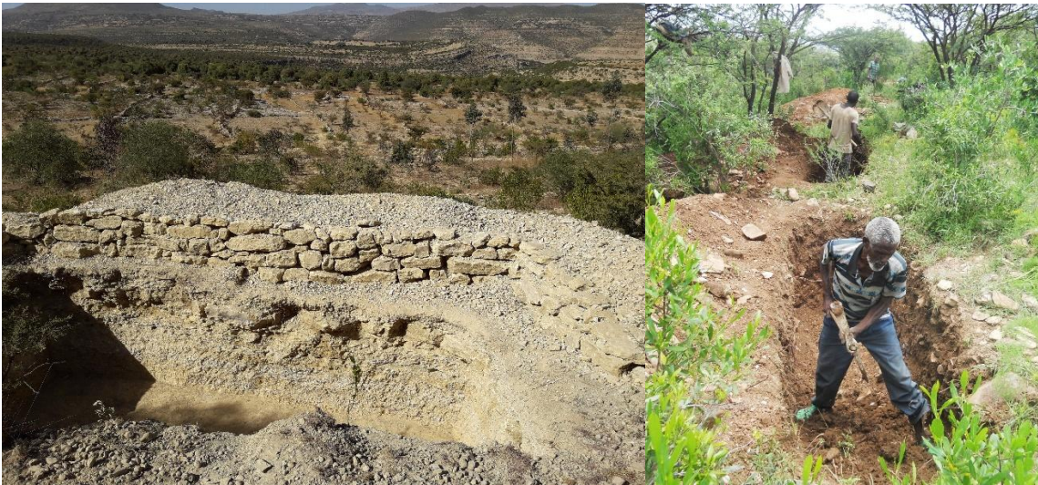
Figure G1.2: Typical examples for project percolation/infiltration pits, assuredly covering well below 10 per cent of the project areas.
