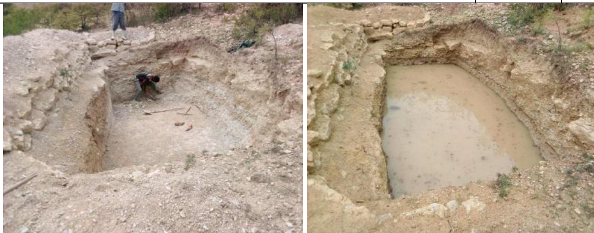
Figure 5 (a – b): Moisture harvesting activities at Meam Atali. EthioTrees started to excavate 2 big (6*3*2 m) percolation ponds and 25 moisture harvesting trenches (3*1*1 m) as moisture harvesting structures in the exclosure.
