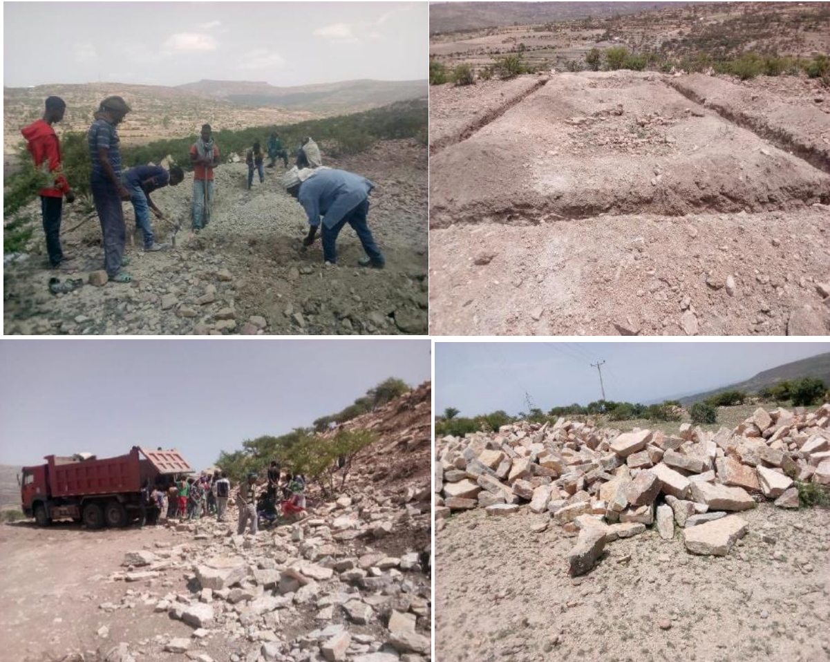
Figure 15. Collecting stone masonry to construct the school and excavation of the foundations.
