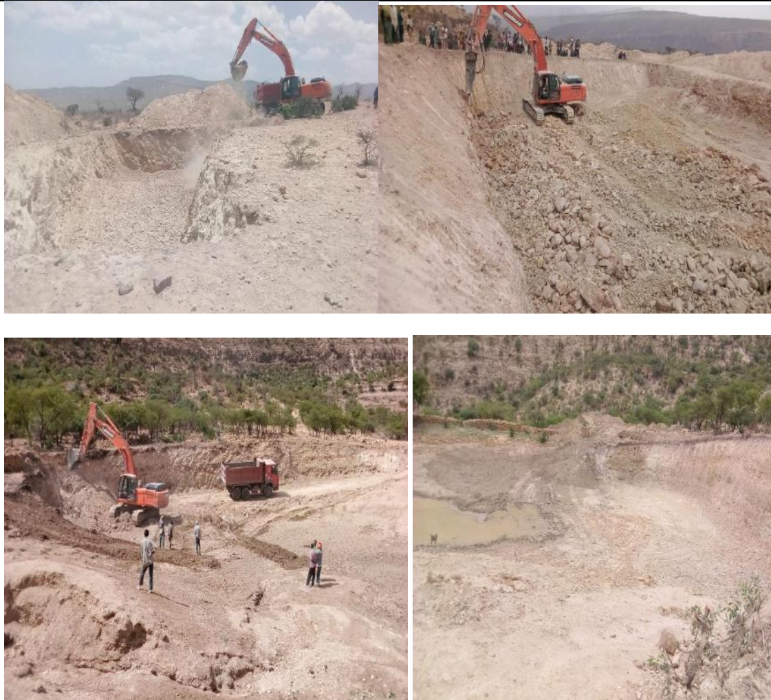
Figure 9: New water reservoirs were constructed in Adi Lihisti village, in Horye Gidimi (40x15x5m), in Meam Atali (expansion with 71.75 m 3 and 105.7 m stone masonry), in Adilal (21 x 18.5 x 3 m), in Mitsilal Aferas (Emnekelelu) (33 x 60 x 1.2 m), and in the village of Walta.
