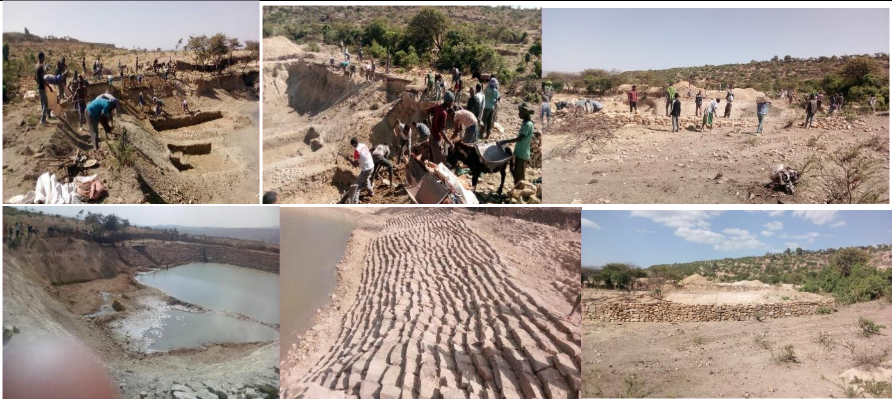
Figure 8: In Adi Keshefo, a new pond was excavated ( 537\text{m}^3 soil was excavated and 192\text{ m}^2 stone masonry wall to support the reservoir).
