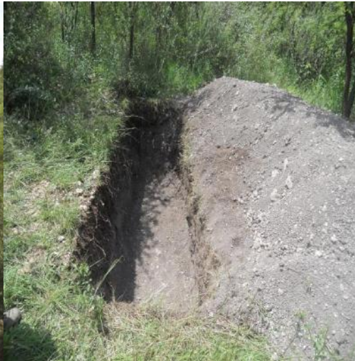
Figure 7: Irrigation trenches at Sesemat (up), Maibaati (middle) and Gemgema (down). About 20-24 percolation ponds were installed at each site – spatially separated as it provides a good advantage to capture the runoff water for infiltration.
