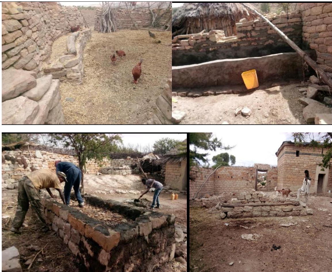
Figure 14: Making a cattle drinking spot near the reservoir of Meam Ataly with supporting cement – in order to save the animal fodder from wastage; and different feeding boxes near the houses.
