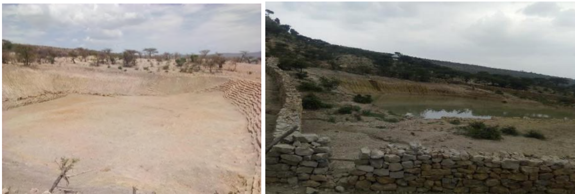
Figure 10 (a & b). Final excavated pond of Hizaty Gidmy, constructed by stone walls with 1 meter height * 0.6 meter width * 188 meter length.
