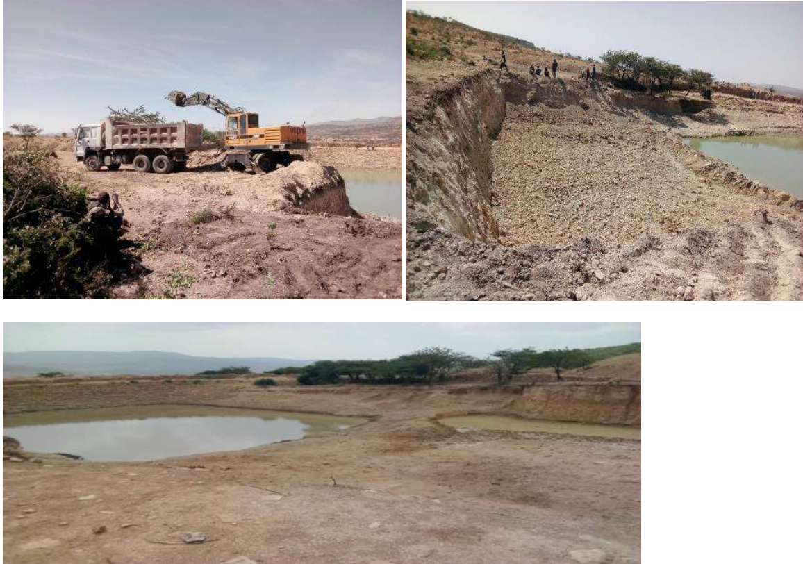
Figure 7 (a -c). Excavation of pond at Adikeshefo.
