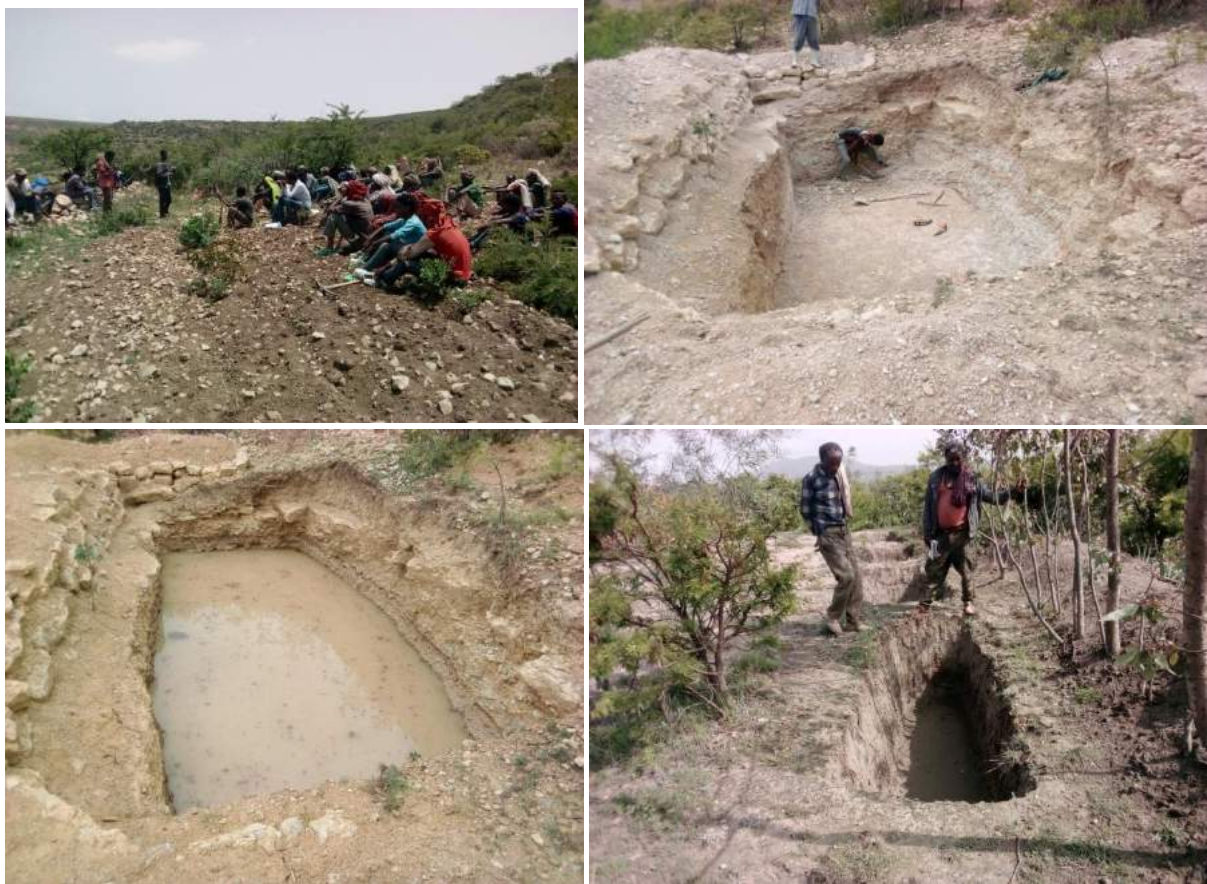
Figure 9 (a – d). Moisture harvesting activities at Meam Atali. EthioTrees started to excavate 2 big (6*3*2 m) percolation ponds and 25 moisture harvesting trenches (3*1*1 m) as moisture harvesting structures in the exclosure.
