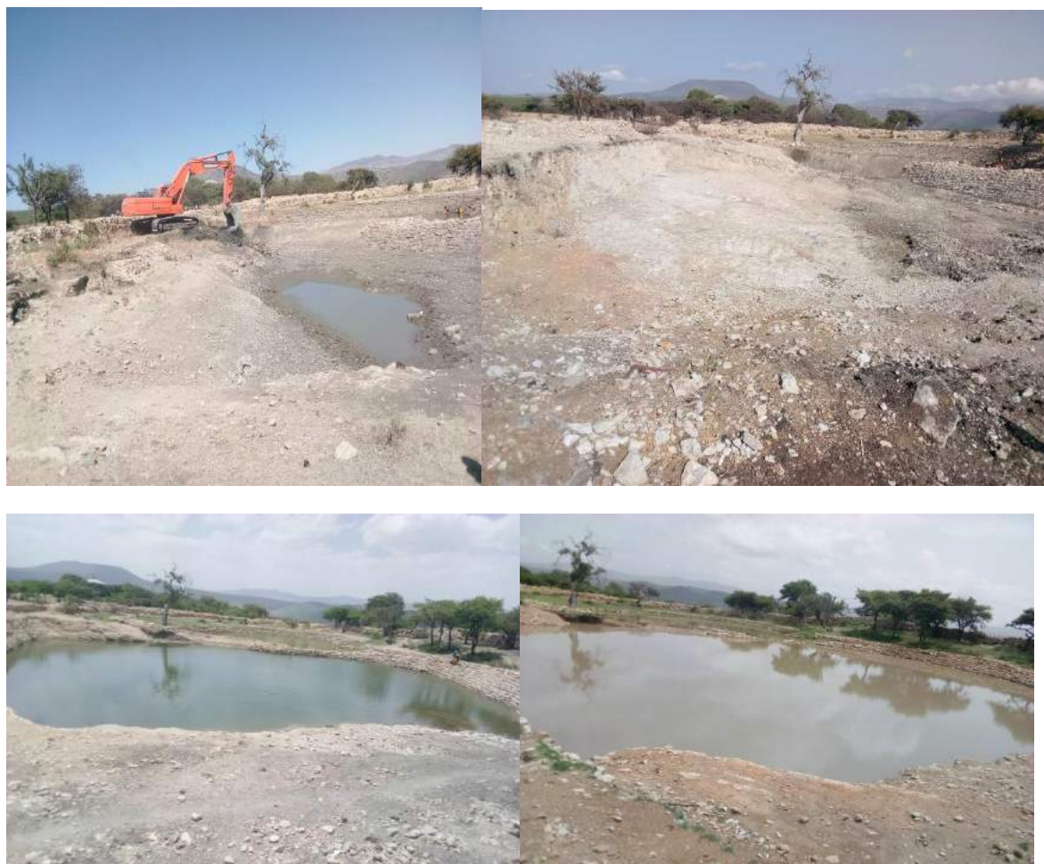
Figure 8 (a - d). Excavation of pond at Adikeshefo. The upper left side is at the start; the upper right side shows the excavation after the works. After some rain and at end of the rainy season, the pond is happily full of water.
