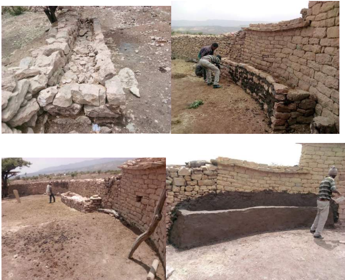
Figure 12. Making a cattle drinking spot near the reservoir of Meam Ataly with supporting cement – in order to save the animal fodder from wastage; and different feeding boxes near the houses.
