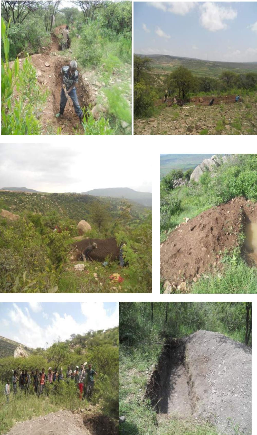
Figure 11. Irrigation trenches at Sesemat (up), Maibaati (middle) and Gemgema (down). About 20-24 percolation ponds were installed at each site – spatially separated as it provides a good advantage to capture the run off water for infiltration.
