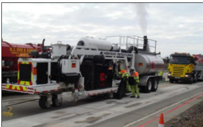
**Figure 1-1 The grinding convoy (grinding machine left, and slurry tanker right)**
