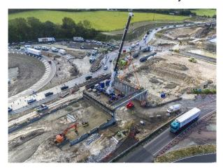
At the end of October, we saw the second big beam lift on the scheme – this time for the northern section of the new flyover.
