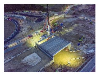
In the centre of Stockbury Roundabout, we've been busy building up the ground level so we can start work on the middle section of the flyover and connect the two bridges that have been built either side of the roundabout. In the finished scheme, this area will see thousands of cars passing over the new flyover every hour.
