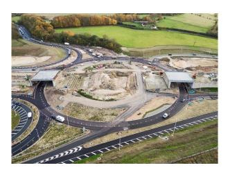
Work has also progressed well on the two bridges on either side of the roundabout. These bridges will take traffic over the roundabout and onto the new flyover and towards the end of the month, we started waterproofing the bridge decks as we continue to get them ready to carry traffic.
