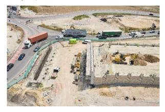
We've also started removing the section of Maidstone Road that has been closed to motorists. This marks the start of the slip road from the A249 southbound to
