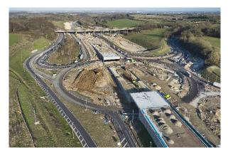
Within the centre of the Stockbury Roundabout, work has been progressing on the new flyover. We've been busy building up and filling the retaining earth (RECO) walls that will support the new road, and allow traffic to pass freely over the roundabout. The last RECO wall is set to be installed in mid-February, marking a huge milestone for our scheme. These flint and cobble clad walls have been specially designed to fit in with the surrounding area of outstanding natural beauty.
