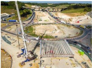
For a week after the bridge beam lift, we had a smaller mobile crane on site to install the concrete panels that fit between the beams.
