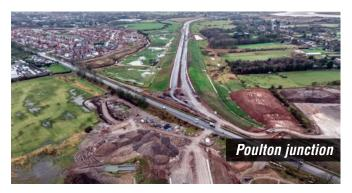
Work at Poulton junction continues to progress. The next stage of work will include installing traffic signals and putting new kerbs and pavements in place.
