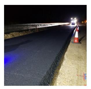
Once the resurfacing is complete, we'll install new kerbs and steel central reservation barriers and add temporary lining in preparation for moving the traffic to the eastbound carriageway, so we can start reconstructing the westbound carriageway.
