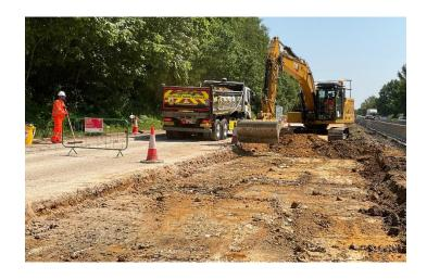
On Tuesday 20 June, we started building the new foundations using strengthened material on lane 2 of the road. Once this work is complete, we'll begin laying the first layer of asphalt surface, before moving to lane 1 to begin rebuilding that lane of the road.
