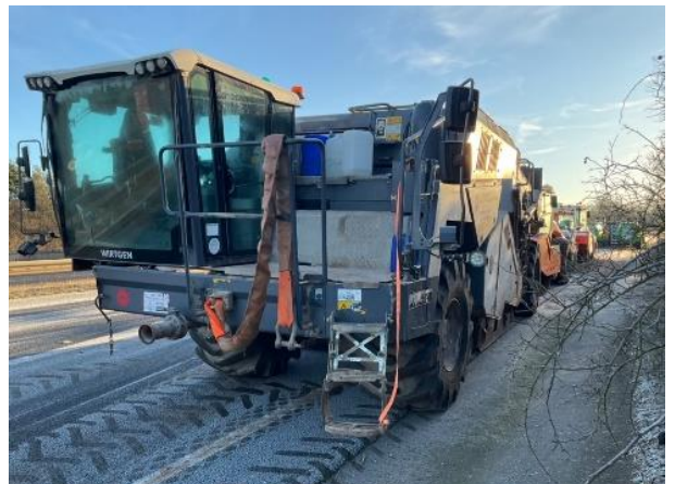
Machinery used to add the strengthening agent
