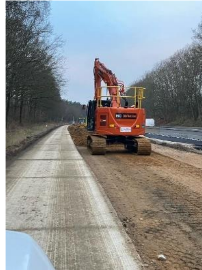
Machinery removing surplus material
