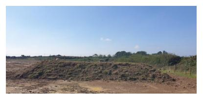
After stripping the topsoil, which will be stockpiled nearby, plastic pipes and wooden boxes, will be arranged in a pattern similar to the tunnels and chambers badgers dig to make a sett. It will be less than 1 m in height, covered with topsoil and seeded for protection from erosion.
