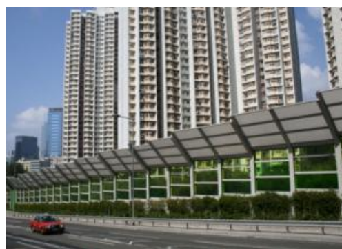
Figure 15. Modified noise walls in Hong Kong
