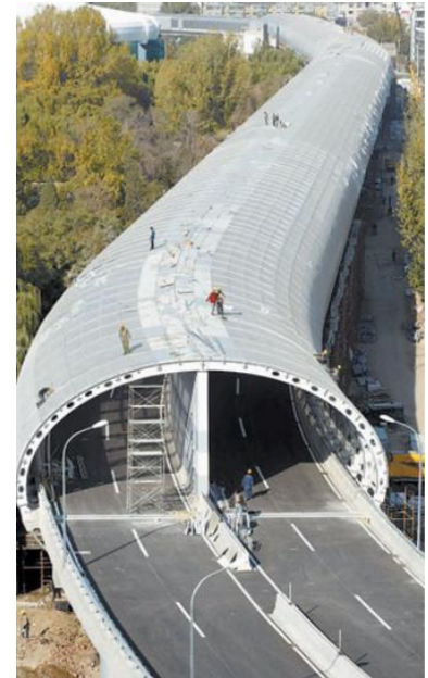
Figure 22. Soundproof tunnel over Beijing Zoo
