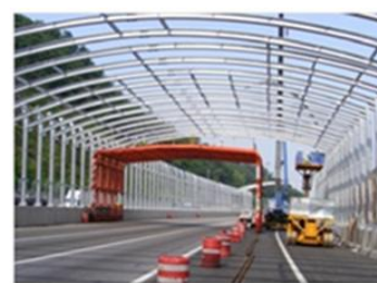
Figure 24. Scaffold arrangement used in South Korea during construction over a live carriageway
