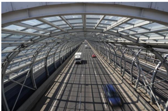
Figure 21. View looking through a soundproof tunnel in Warsaw
