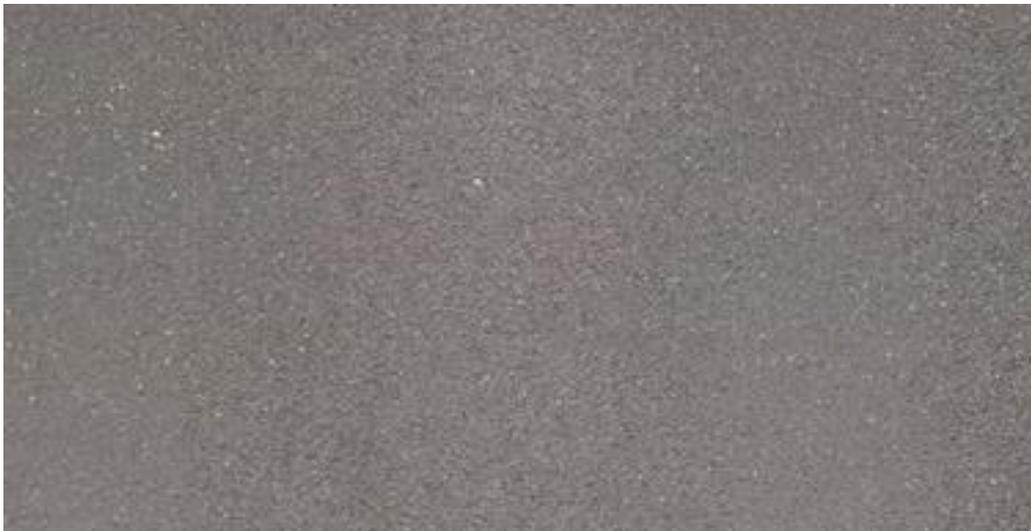
Figure 13: Loss of Aggregates/Fretting (f)
