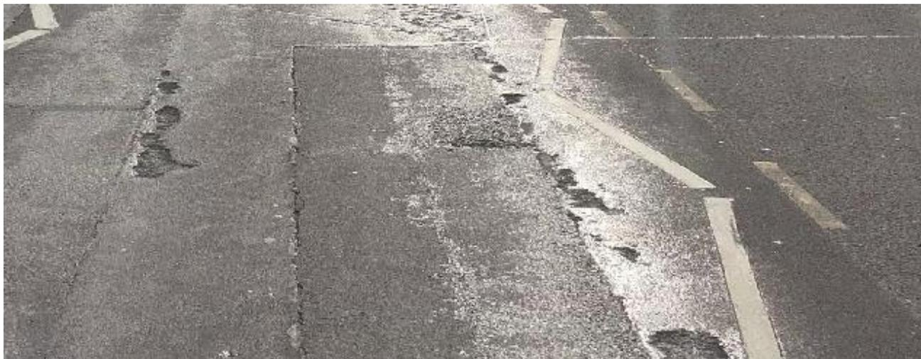
Figure 9: Variable Defects (v) including Potholes (p)
