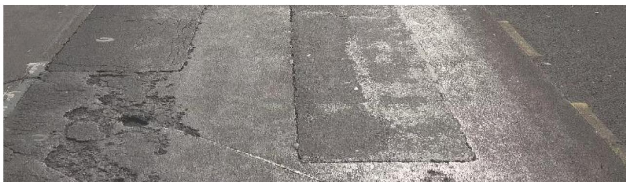
Figure 8: Loss of Aggregates (-) and Evidence of Pothole Formation (p)
