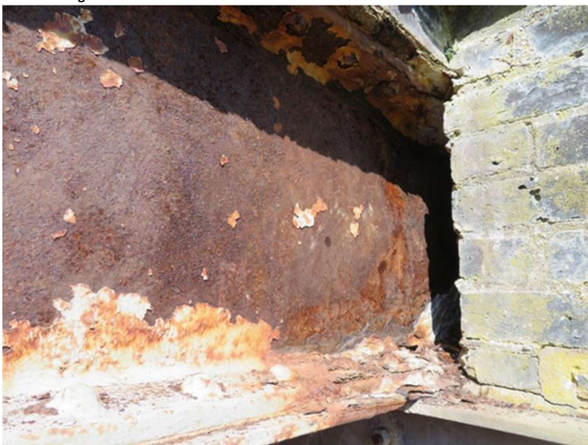
Southern edge girder, eastern end support.
