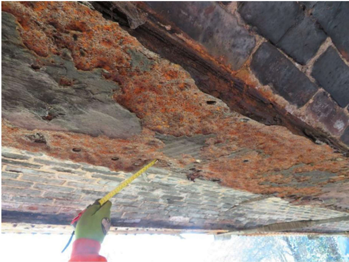
Southern internal beam soffit.
