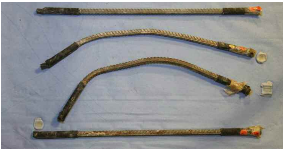
Figure 22: Top surface of bars removed from Specimen 1A
