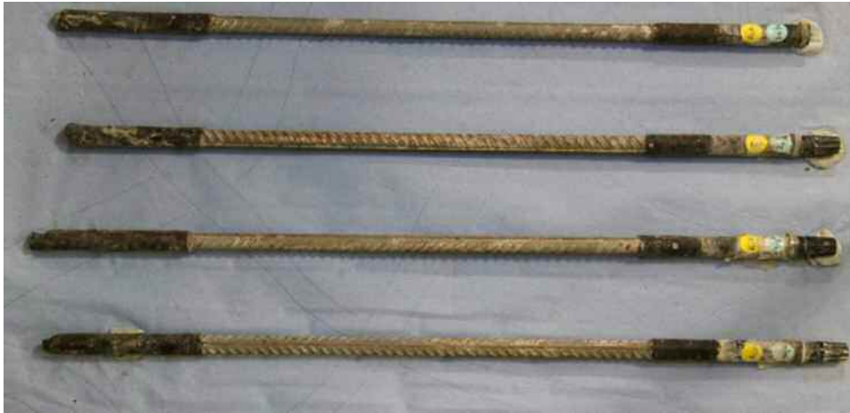
Figure 30: Top surface of bars removed from Specimen 24A
