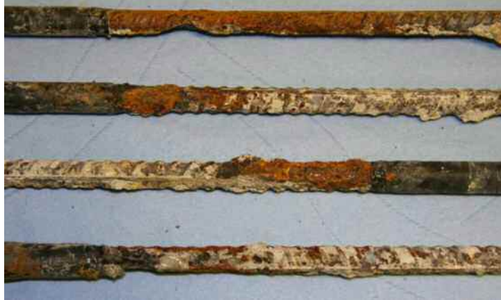
Figure 13: Close up photograph of bars removed from natural aggregate specimens
