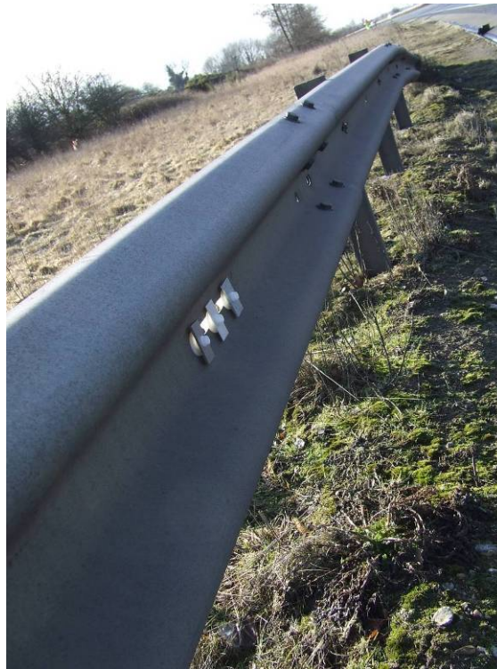
Plate 2-5 Fixing detail on TCB
