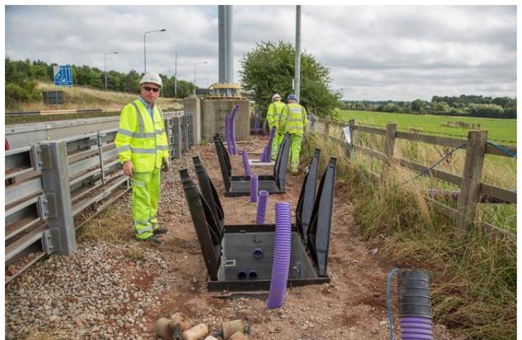
Ducts being checked in the verges prior to the installation of cables
