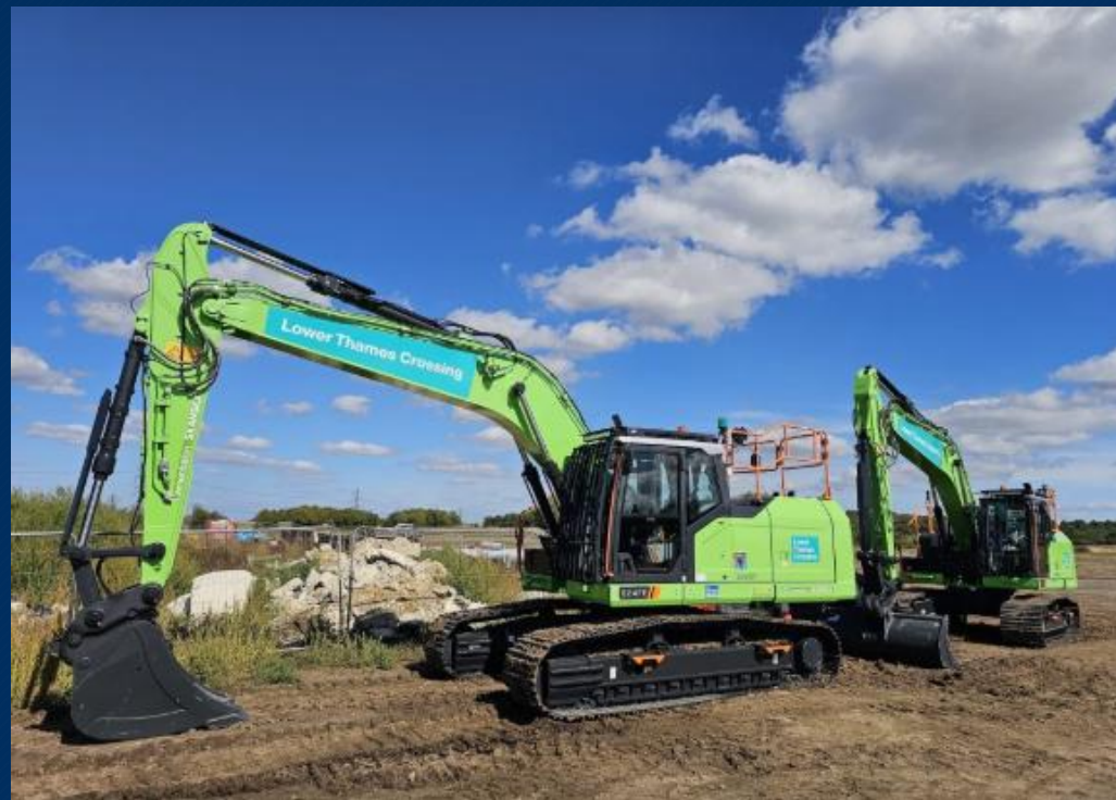
Two excavators – to be named by Thamesview School
